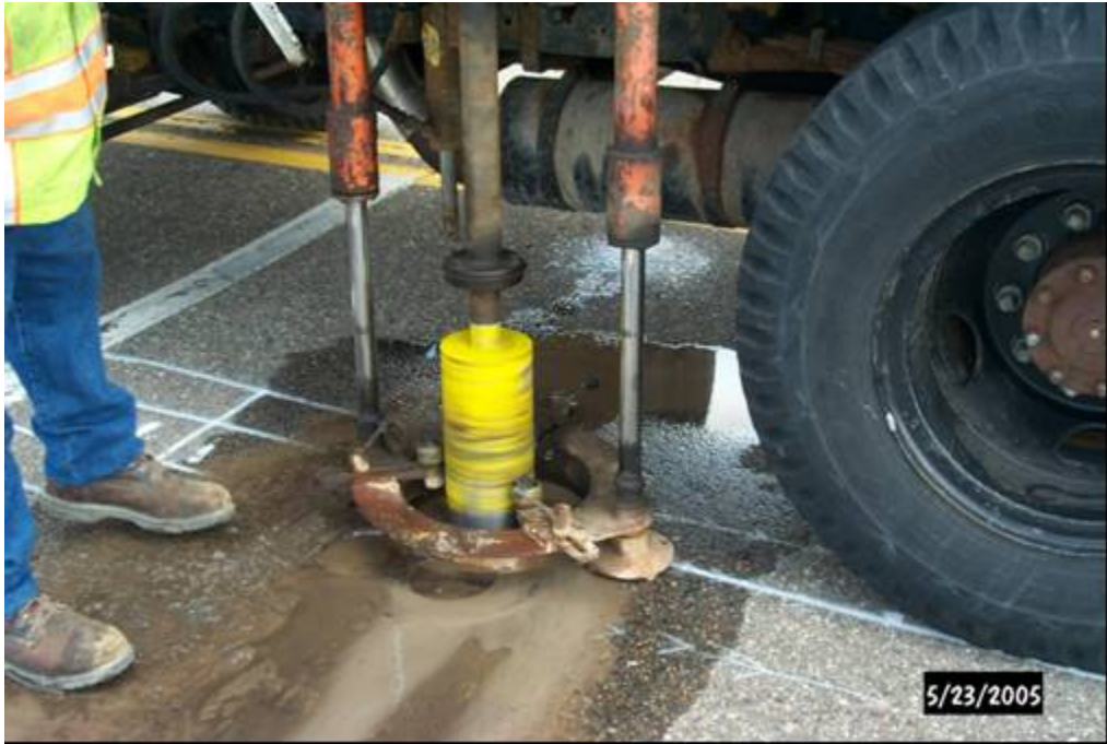
Figure C-2. Coring with core truck
