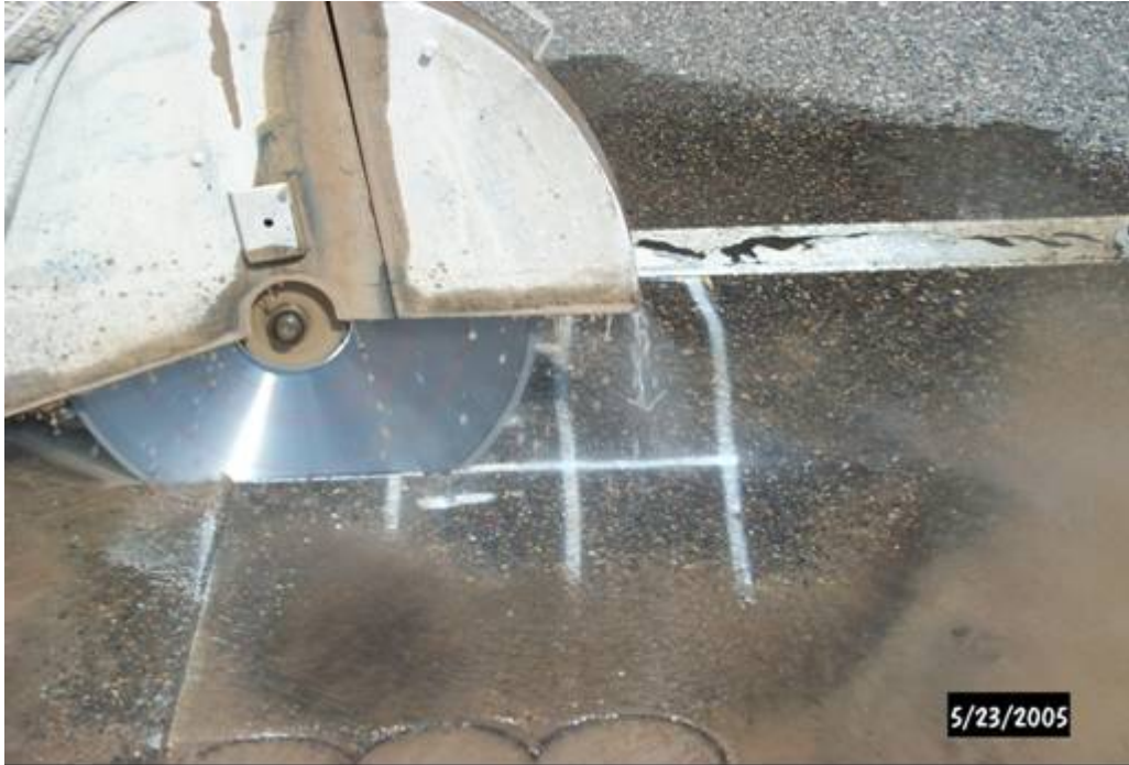
Figure C-3. Saw cutting beam samples
