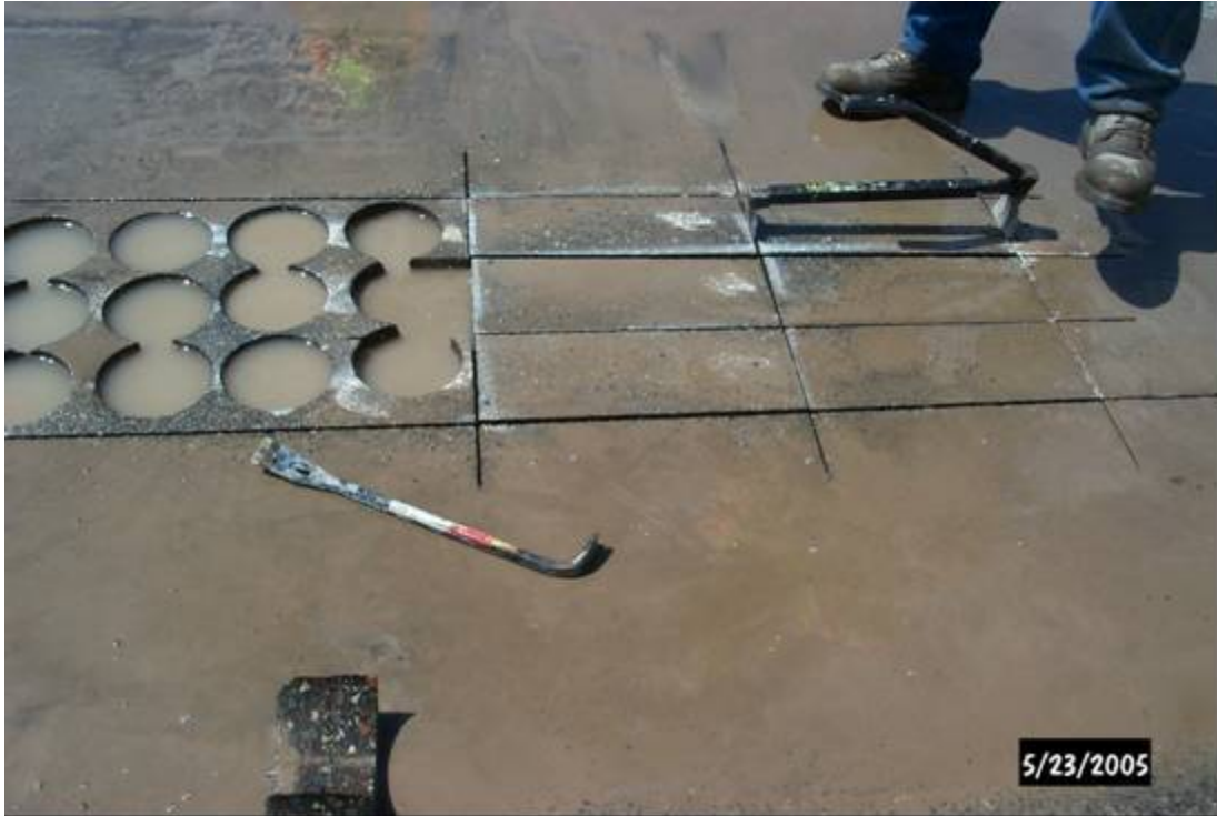
Figure C-5. Sample area and tools for removing beams
