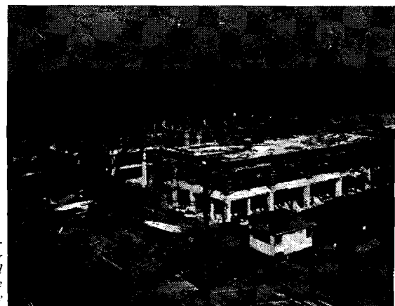
A corner of the Library as it was two years ago. This shows the skeleton steel and concrete construction that was used.
