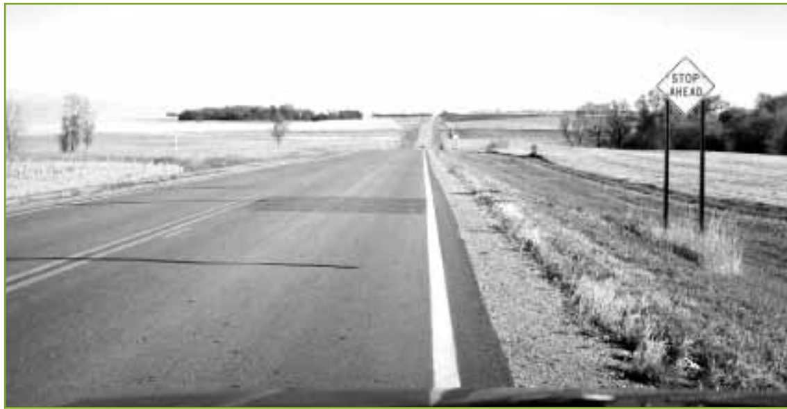
Rumble strip and warning sign in Lincoln County
