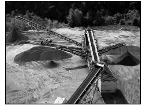
RAP segregated in piles
