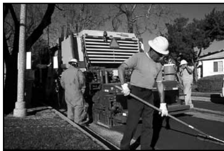
Rubberized slurry seal in Los Angeles
