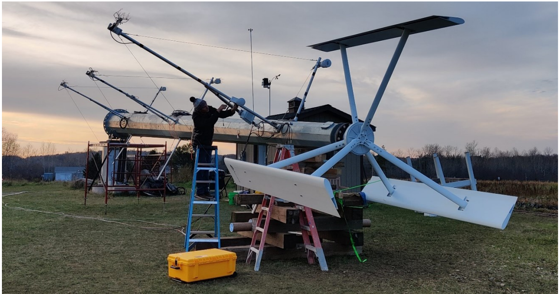
Figure 1.2: Tower lowered for installation of the turbine and sensors.
