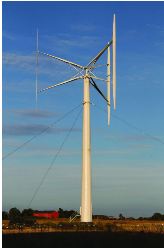
Figure 1.19: 200kW T1-turbine by Vertical Wind AB and Uppsala University from (Möllerström et al., 2016).
