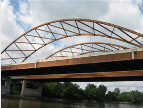
The Cedar Avenue Bridge in Burnsville, MN
