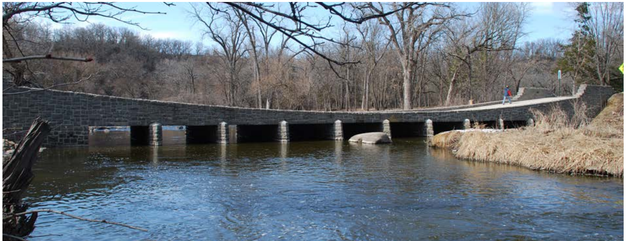
Redwood County's swayback bridge features an overflow section for high flows.
