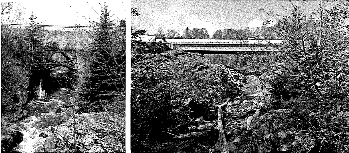
Figure 2. Example modification of a bridge to encourage wildlife use of an underpass. On the left is the original bridge, on the right is a widened bridge span with room for animals to cross underneath. Photo credit: Mn/DOT.
