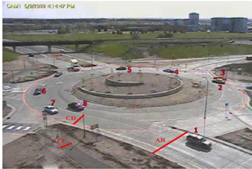
Figure 2- 4. An image of the roundabout.
