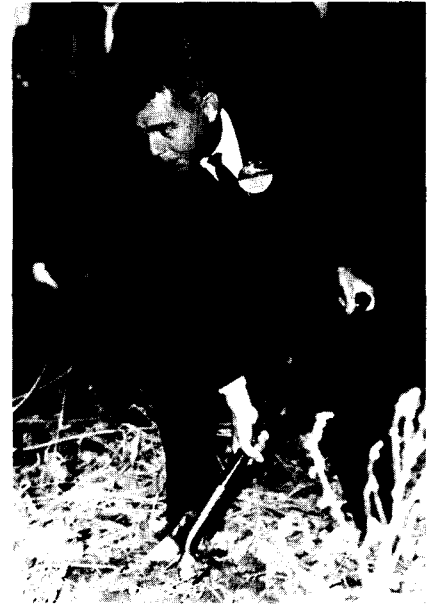
Dean Rodney A. Briggs turns the first shovelful of earth at ground-breaking ceremonies for UMM's first new building—a 120-student residence hall.
