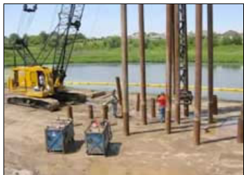
Workers drive piles to support a roadway expansion
