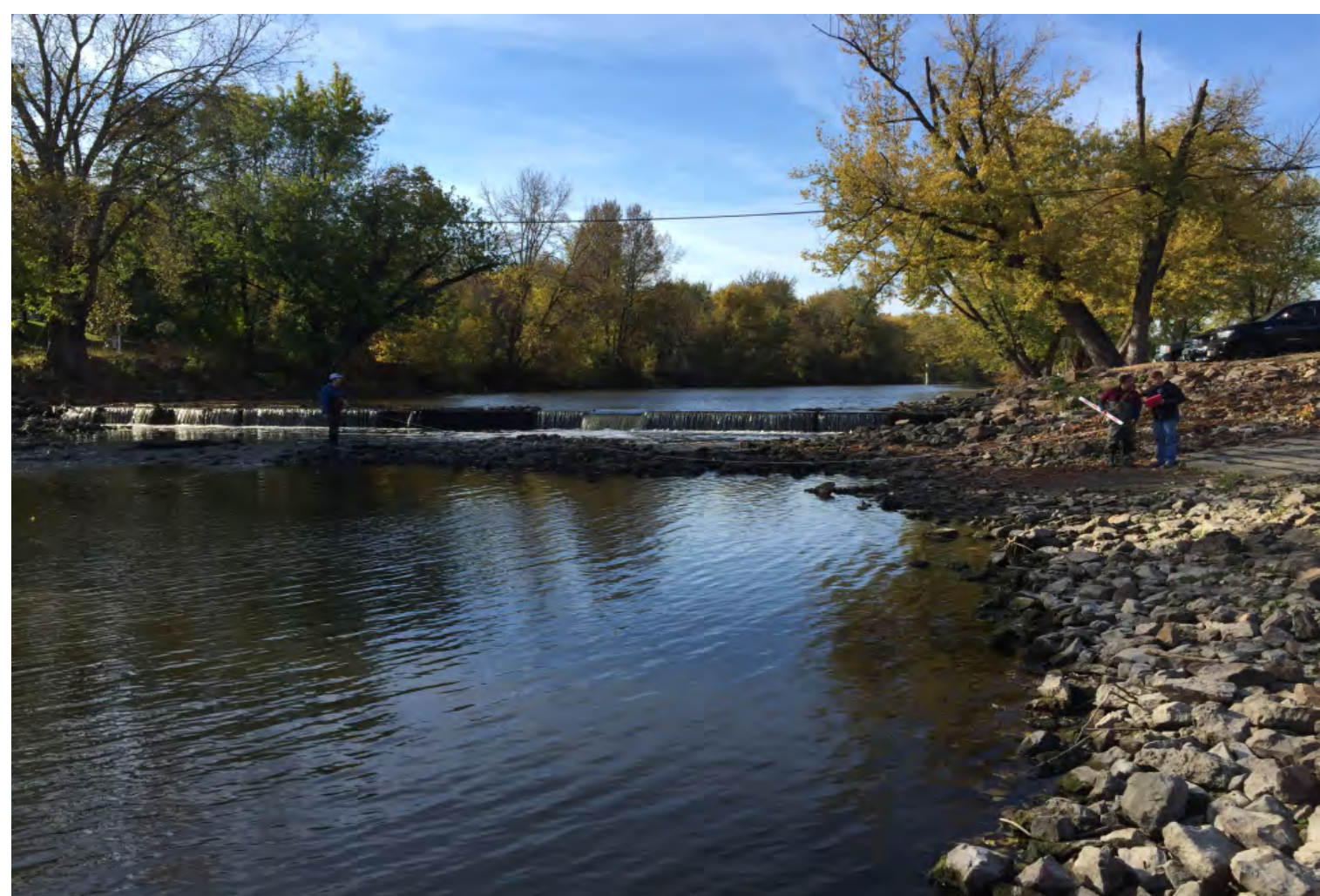
Current condition of the Watertown Dam in 2015. By: Garcia-Serrana, M.
