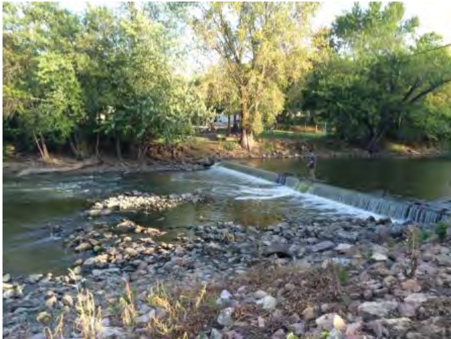
Figure 5. Current condition of the Watertown Dam in 2015.
