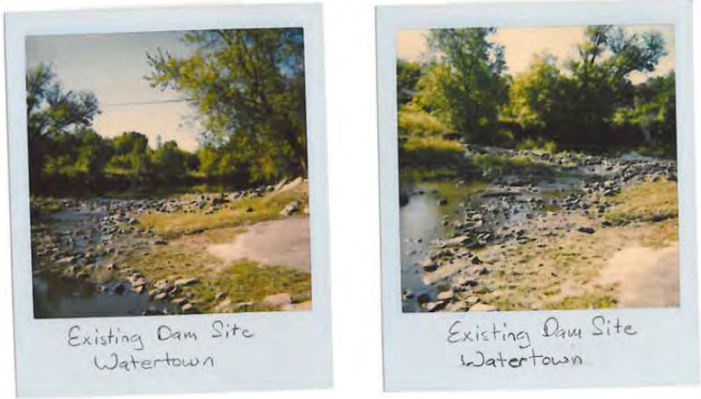
Figure 1. Existing Watertown Dam, prior to the 1988 reconstruction.
