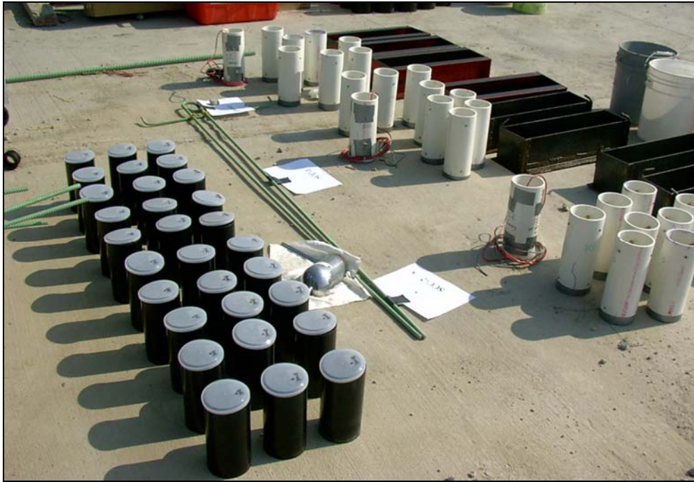
Figure D-1 Companion concrete cylinder and modulus of rupture beam forms in the field
