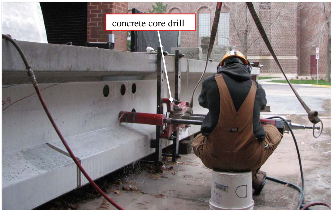
Figure D-6 Setup for taking concrete cores
