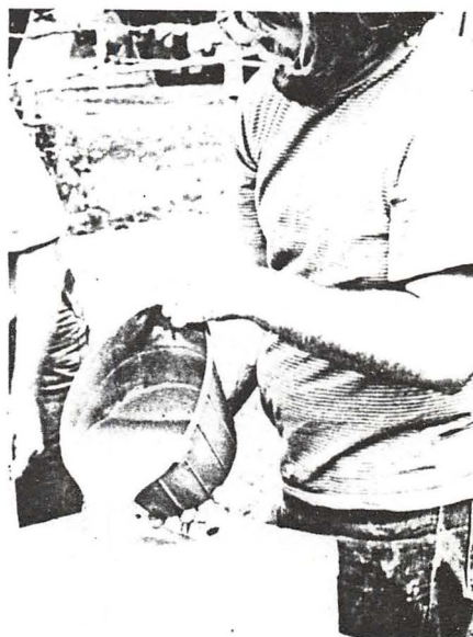
(14) Pouring liquid clay slip onto plaster to stiffen.
