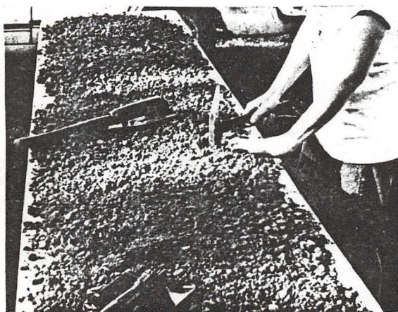
(13) Drying and pulverizing clay.
