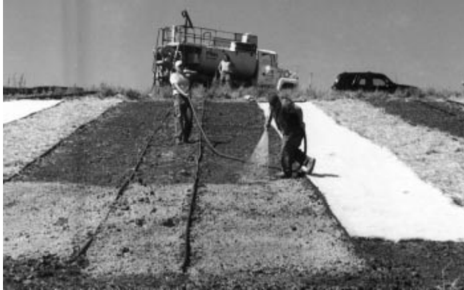
Figure 2.8. Application of Sprayed Emulsion Product.
