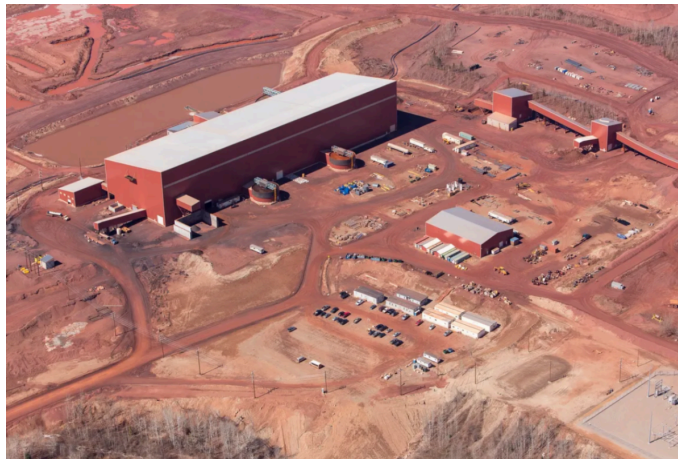
MagIron LLC Plant 4, in Bovey, Minn., near NRRI's Coleraine facility.
