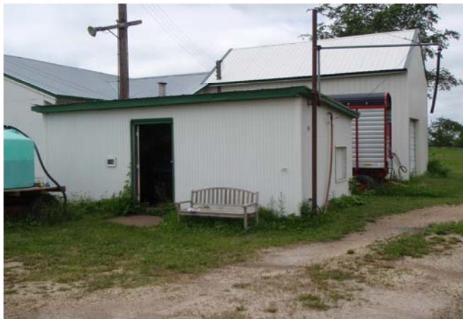
Pump House for Well 207617
