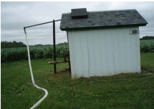
Pump House for Well 207608
