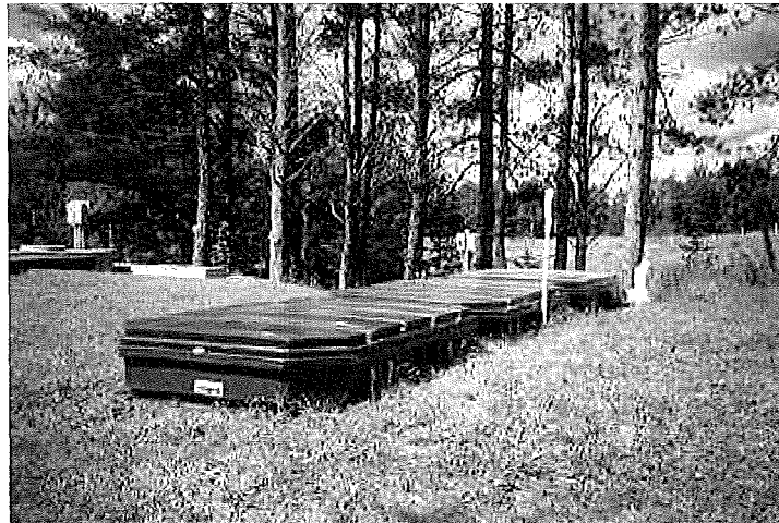
Photo 5. Completed Puraflo® system (3 modules).
