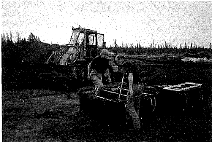
Photo 1. Placement of Minnesota peat medium at MSI.
