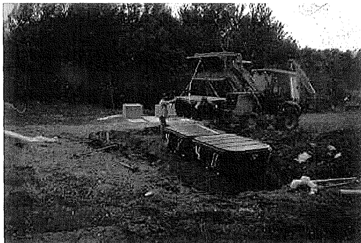
Photo 3. Module placement in level excavation.
