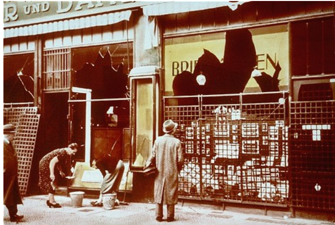
Storefronts of Jewish-owned businesses damaged during the Kristallnacht ("Night of Broken Glass") pogrom. Berlin, Germany, November 10, 1938. - Bildarchiv Preussischer Kulturbesitz USHMM
