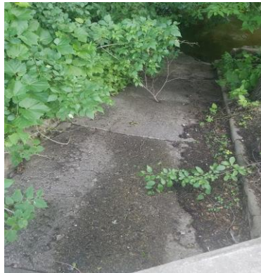
Figure 2.22 - Sloped Concrete Impervious Surface Leading Down into Minnehaha Creek.
