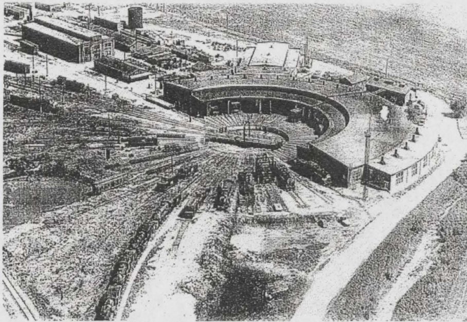
A round house similar to the one below once occupied the space in the center of the present era photo at right. Round houses provided maintenance to steam locomotives between runs and were equipped with a turntable (center) which was used to redirect them to the track of their next assignment. (They were also, according to Watty Piper, social places, where engines could go when they were not busy.)
