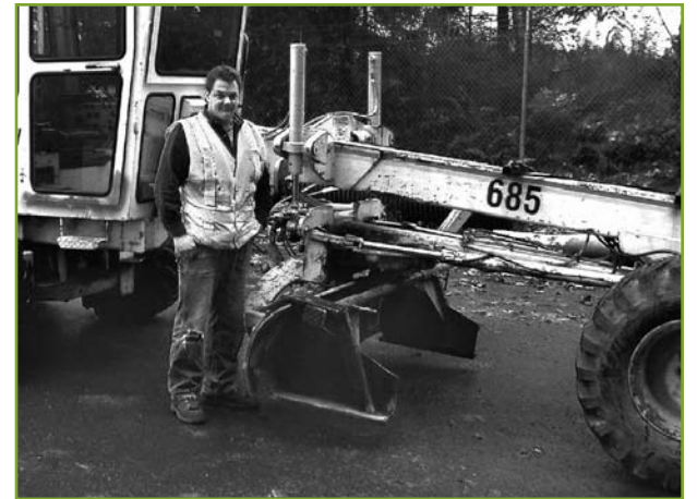
The two “boots” are width-adjustable for patching.
