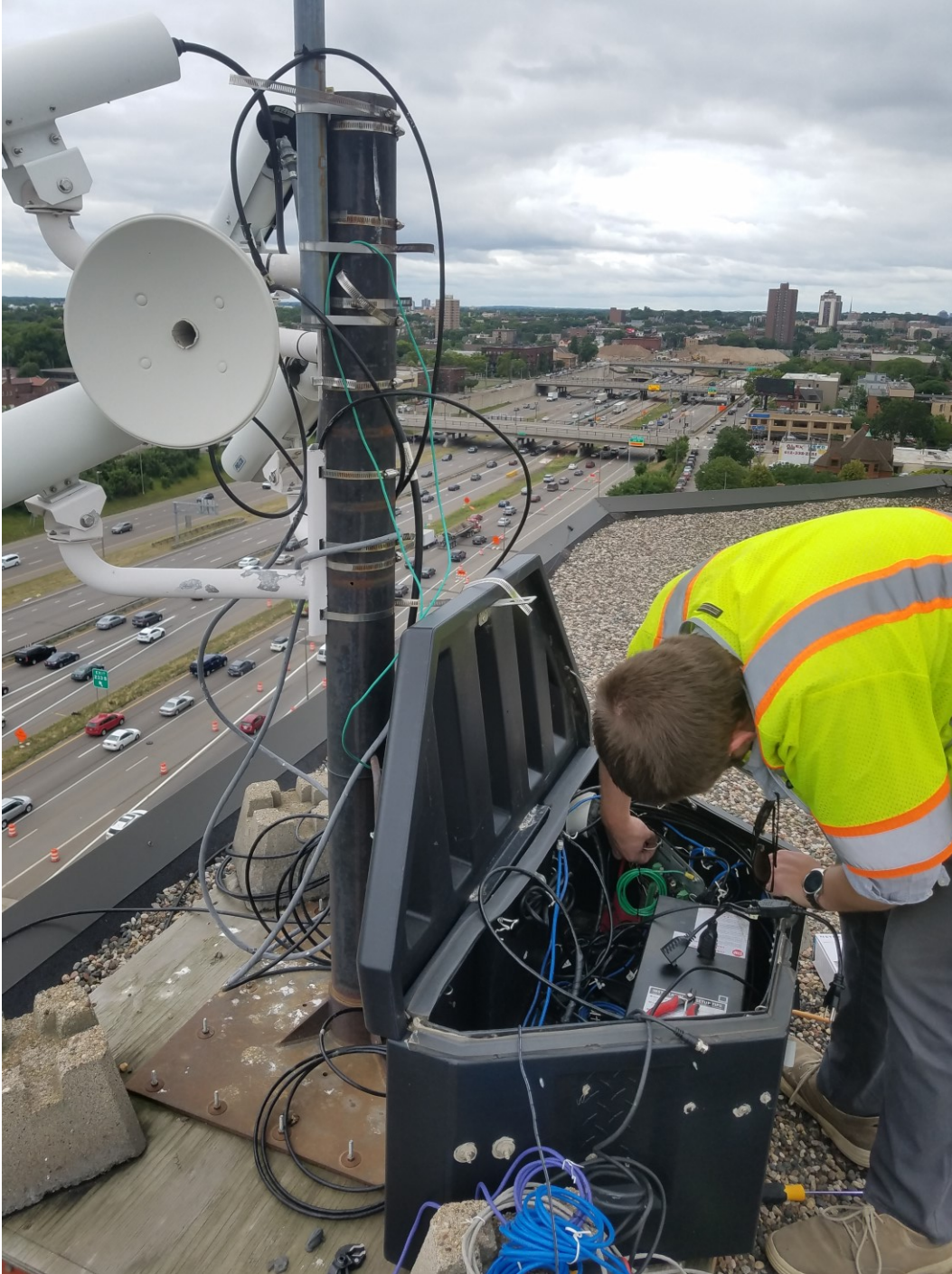
Figure 2.7 MTO engineer Gordon Parikh repairing the Augustana station
