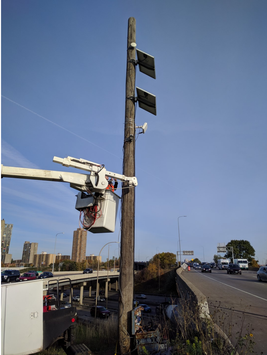
Figure 2.3 Hiawatha station being assembled.
