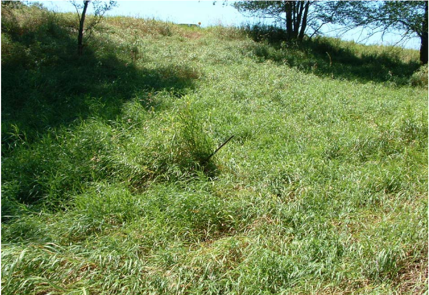
Photograph 08: Example Rebar Protruding in 154 th Street Disturbed Area
