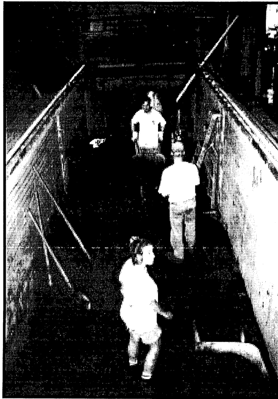
Photo 1. Placing soil in channel.
