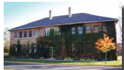
Originally completed in 1901, the Veterinary Anatomy building was vacated in 1996.
