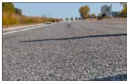
Porous asphalt test cell on the MnROAD LVR
