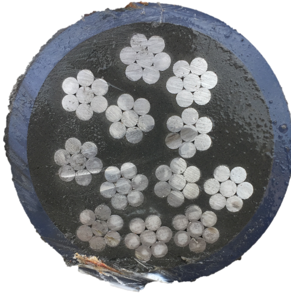
Figure 2.7 Tendon adequately full of grout
