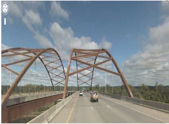
(a) Photograph of the Bridge
