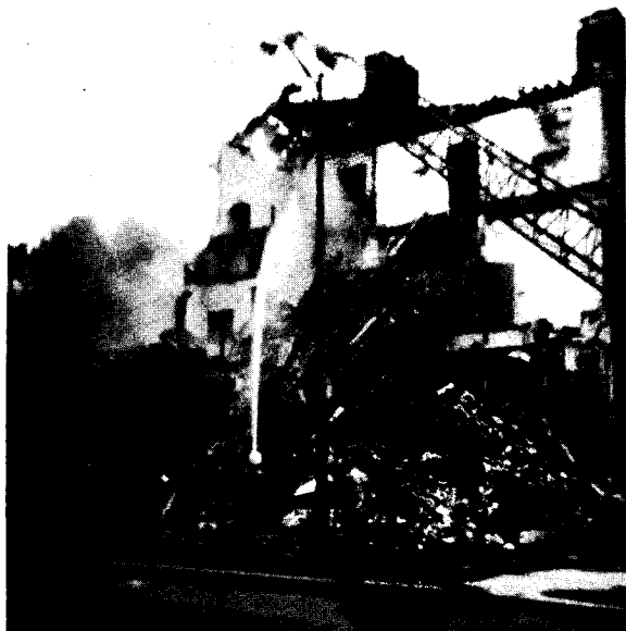
Tearing Down the Agricultural Botany Building (Tottering Tower)
