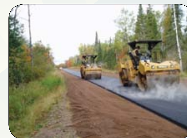
Lake County saved about 19 percent on the non-wear and 4 percent on the wear mixture by using high percentages of RAP.
