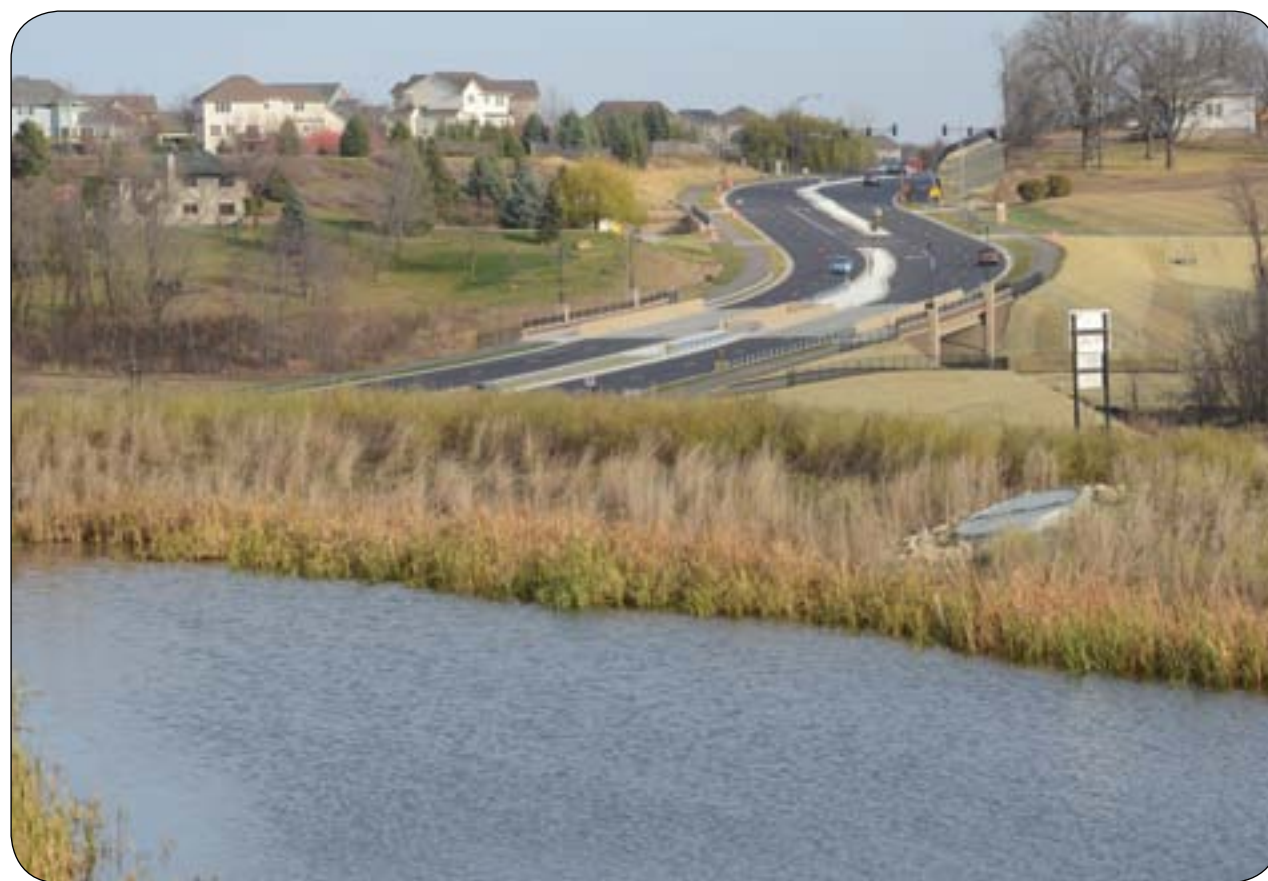
The Bass Lake Road Reconstruction Project minimized impacts to natural and historical features.
