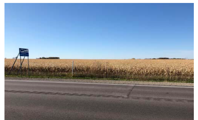
Researchers tested samples from an asphalt pavement on State Highway 22 that included J-Band under the longitudinal edge joints of asphalt lanes.
