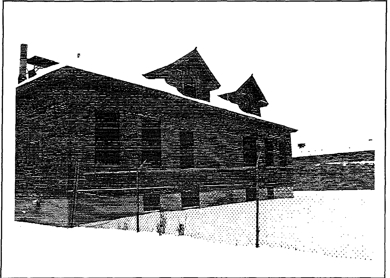
Plate 6: Building #250, the District Chem Lab, December 1996. Photo by Patrick Nunnally, from the collections of the Minnesota Historical Society.
