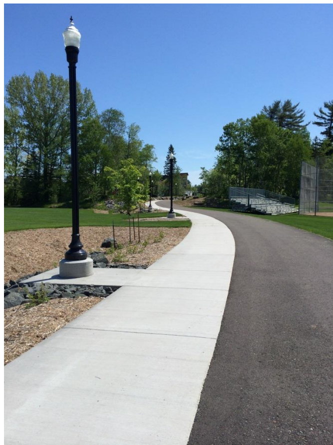
The completed pathway connecting UMD to BlueStone Commons. Contributed Photo
