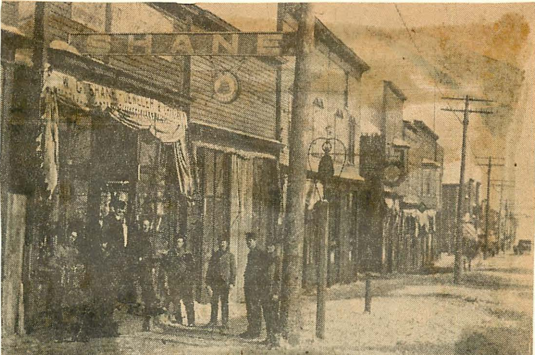
REBUILDING CREW —Pictured is the telephone men who rebuilt Chisholm's telephone system after the great fire of 1908. The poles, cable and wires shown in the picture were part of the telephone plant entirely destroyed by fire.
