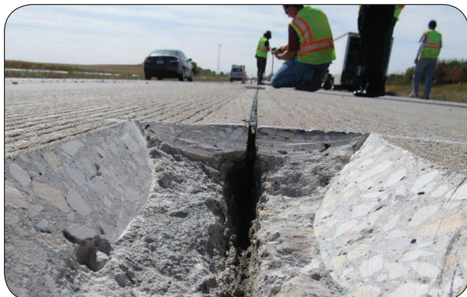
A repair in progress along a distressed/deteriorated joint
