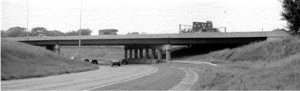
Figure 2.4 Mn/DOT Bridge No. 27734
