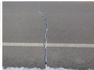
Left: The disk-shaped compact tension (DCT) test for determining thermal cracking potential of asphalt mixes; Above: Thermally induced crack in North- Western Minnesota
