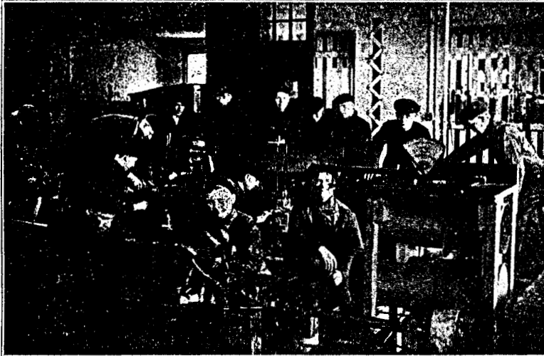
REPAIRING AND OVERHAULING GAS ENGINES AT NORTHWEST SCHOOL
