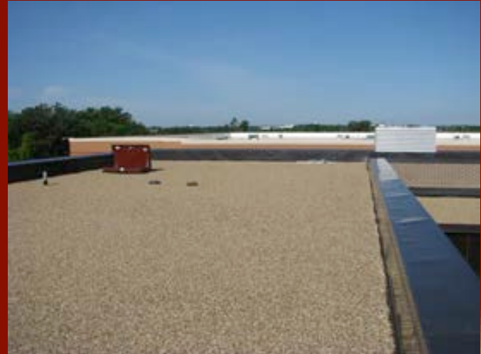
Upper level roof
