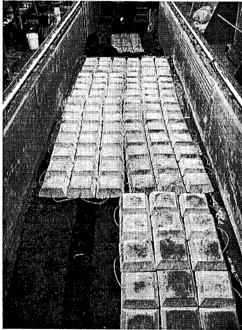
Photo 1. Installation of CC 35 System prior to testing.
