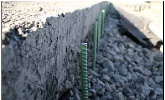
Pervious concrete pavement research at MnROAD
