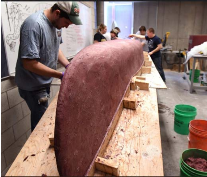
ASCE members casting the concrete canoe
