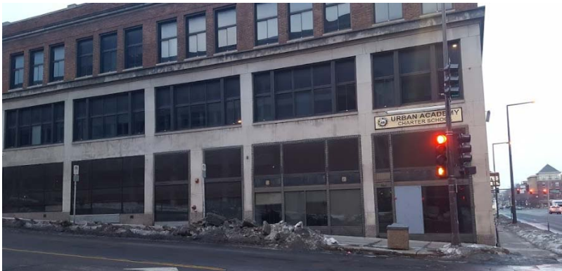
Image 8: Seventh Street East and Robert Street North
