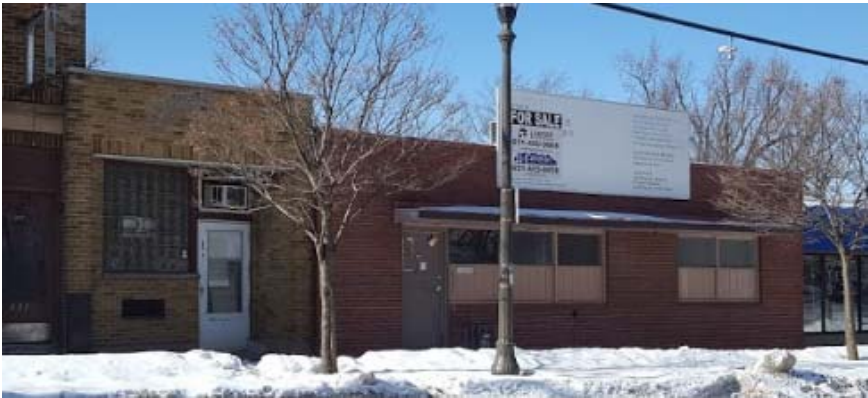
Image 1: South Stryker Avenue near Elizabeth Street West
