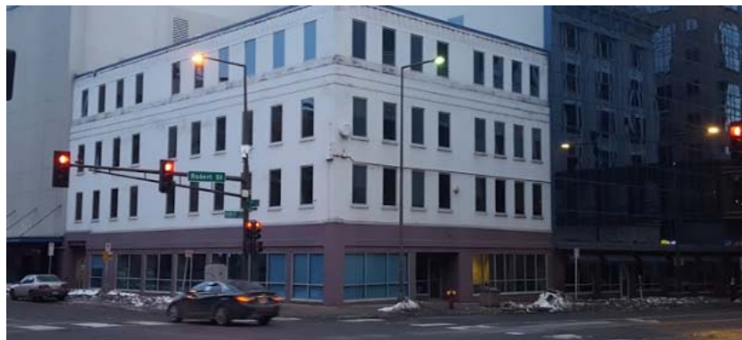
Image 9: Seventh Street East and Robert Street North
