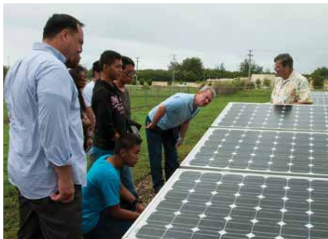
Figure 2: Tour of ground-mounted solar panel.
