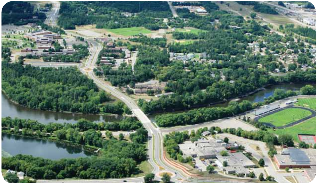
Design elements in the College Drive Reconstruction in Brainerd included three roundabouts, bridge deck modifications to allow pedestrian and bicycle facilities, and storm sewer improvements.
