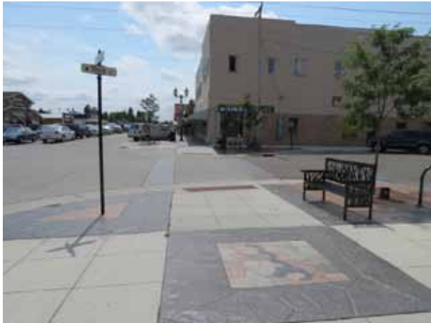
Figs. 4 and 5: Colored concrete for aesthetic purposes and to delineate a path
