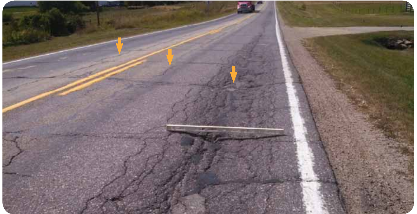
Types of pavement cracking failures, left to right: longitudinal, thermal or reflective, and fatigue
