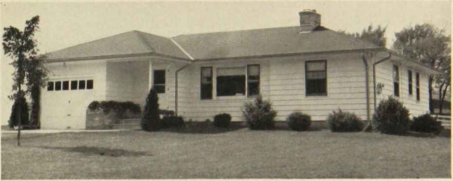
Fig. 2. The one-level and split level type homes suggest greater freedom of design.
