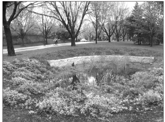
This rain garden was installed on Gortner Avenue in St. Paul to help manage stormwater while improving campus sustainability.
