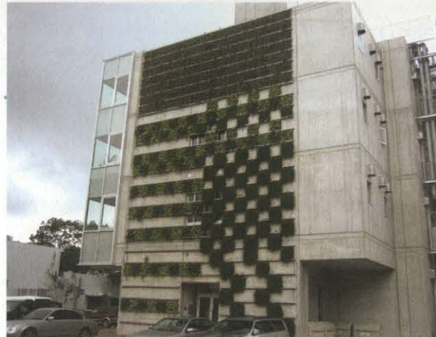
"Tooling with Mother Nature," an article by Blaine Brownell (Arch) in Discover magazine, featured use of Shimizu Corporation's Parabienta building afforestation system.
