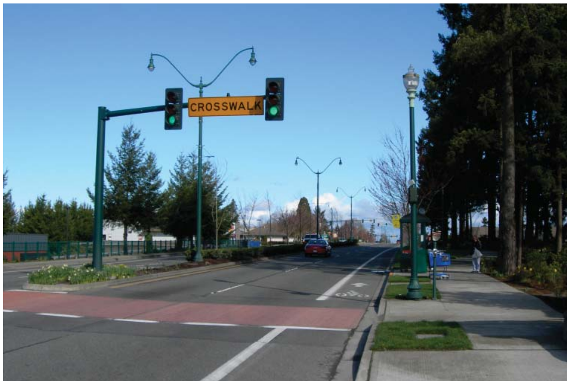
On Bridgeport Way, two mid-block crossings are provided in high traffic areas near an existing commercial area and a planned town center in University Place.
