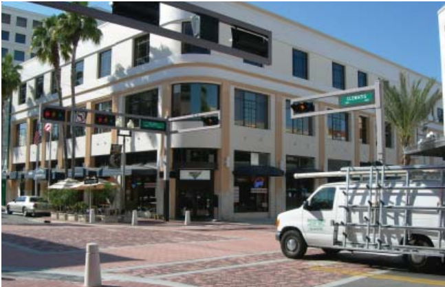
Top: A number of neighborhood traffic calming treatments were implemented throughout the city of West Palm Beach in response to community requests to deal with cut-through and slow down vehicles. Bottom: Downtown traffic calming efforts in West Palm Beach included paved intersections, landscaping, bollards, bumpouts, and improved signage. The streetscape planning and design was facilitated through the Downtown Master Plan process.
