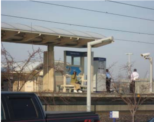
Top: New mixed income housing has been developed adjacent to the transit station. Bottom: The Emerson Park transit station provides an important transportation link for neighborhood residents. (Photo source: Ann Forsyth)
