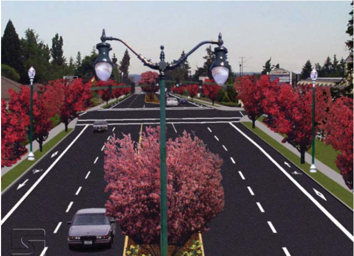
Visualization of proposed enhancements on Bridgeport Way in University Place, WA, was key to allowing participants to understand how existing conditions (as shown in the photo above) could be modified to include the landscaped median and boulevards, multi-modal enhancements, lighting, and roadway alignment. These features are illustrated in the lower photo through computer generated visualization. (Photo source: City of University Place)
