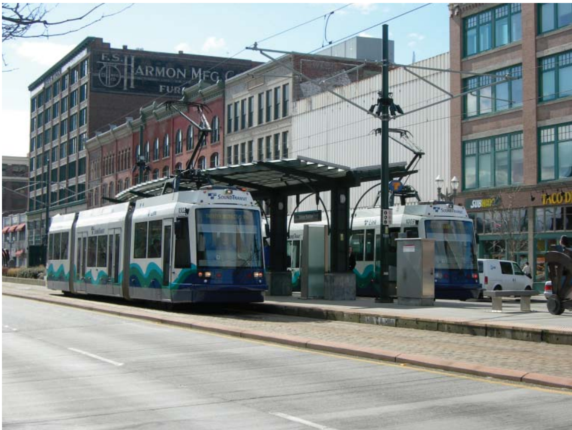
Transit oriented redevelopment near the University of Washington's satellite campus in downtown Tacoma.
