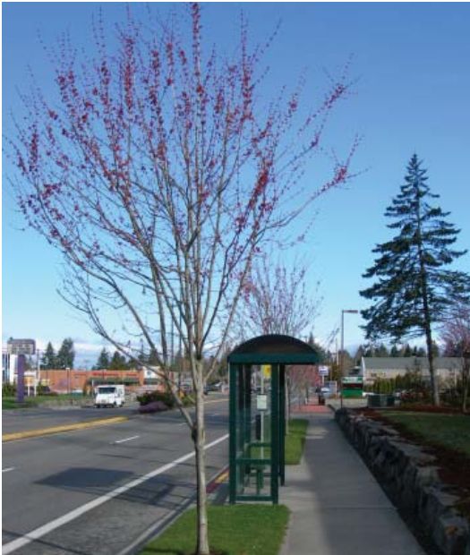
Multi-modal improvements were added throughout the Bridgeport Way corridor in University Place, Washington.
