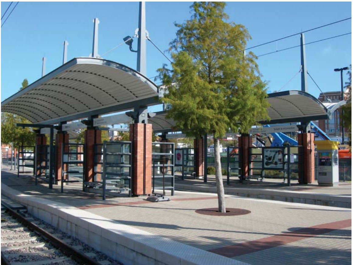
Commuter rail station in Fort Worth, Texas.
